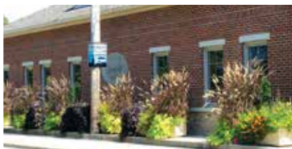
Admin Building "After"
