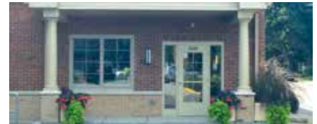
Admin Building "After"
